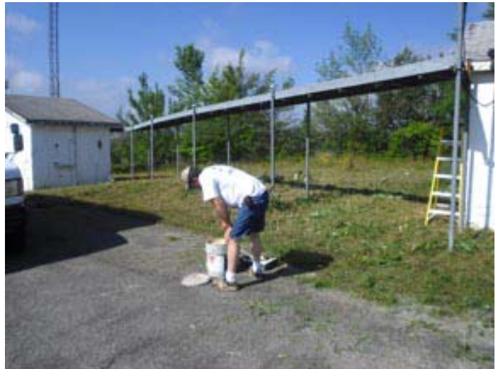
Mark, KC2JNI getting the paint ready to spread.
