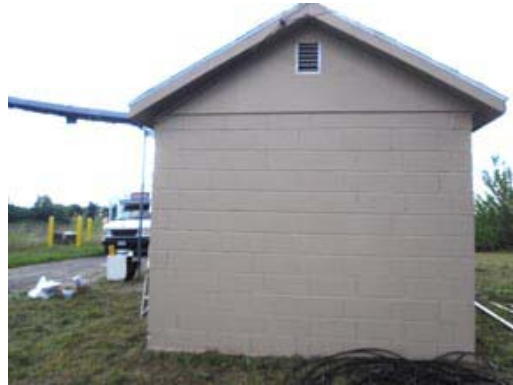
Nice paint job.
